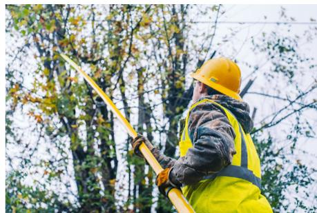
A right-of-way worker cuts away tree limbs and other vegetation that can cause power outages, especially during high winds and storms.
